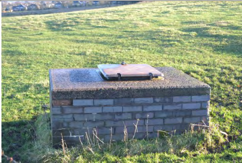
Photograph 4 (facing E): Valve chamber on water main crossing the site.
