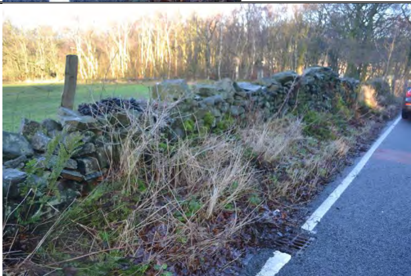
Photograph 3 (facing NW): Gully on Gib Lane likely to connect to culvert crossing the lane to cross the plot.
