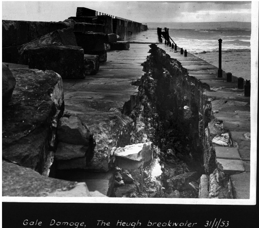
Figure 2: Overtopping damage to the Heugh Breakwater caused during the North Sea Storm Surge of 1953.
