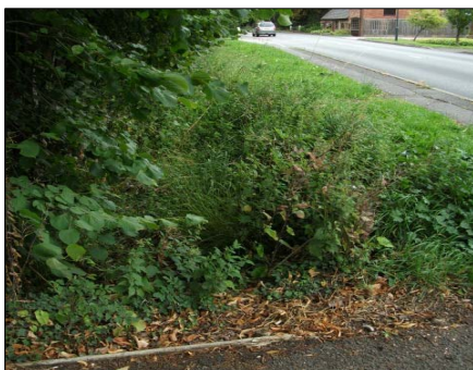
Photograph 6: Poorly maintained drainage ditches
