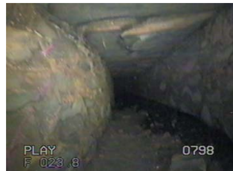
Figure 3- Typical Partial Roof Collapse
