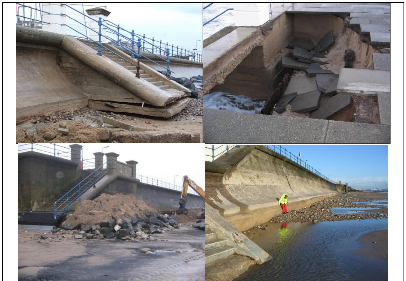
Recent damage and undermining sustained at the coastal defences in Seaton Carew.
