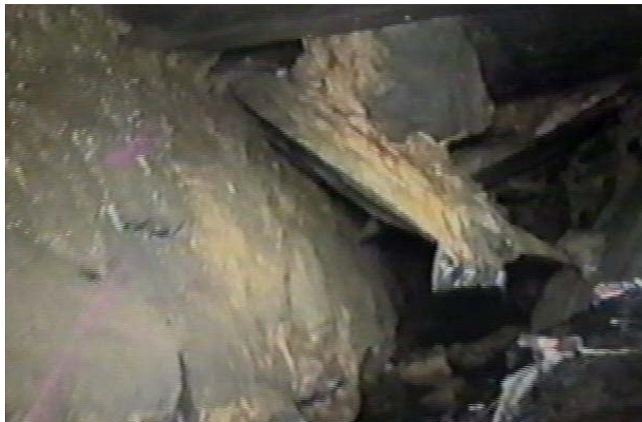
Fig 1 : Collapsed culvert under Leicester road
