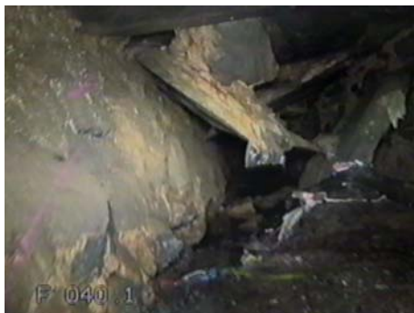
Figure 2-Typical Roof Collapse
