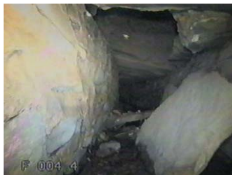
Figure 4 -Complete Roof Collapse
