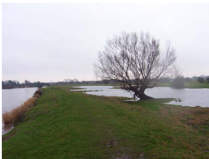
Off-line storage on the Trent, near Rolleston (Notts) during a small flood event; note the River Trent on the left and water in storage on the right.
