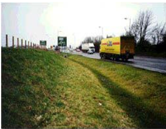
A roadside soakaway; an example of the application of SuDS.
