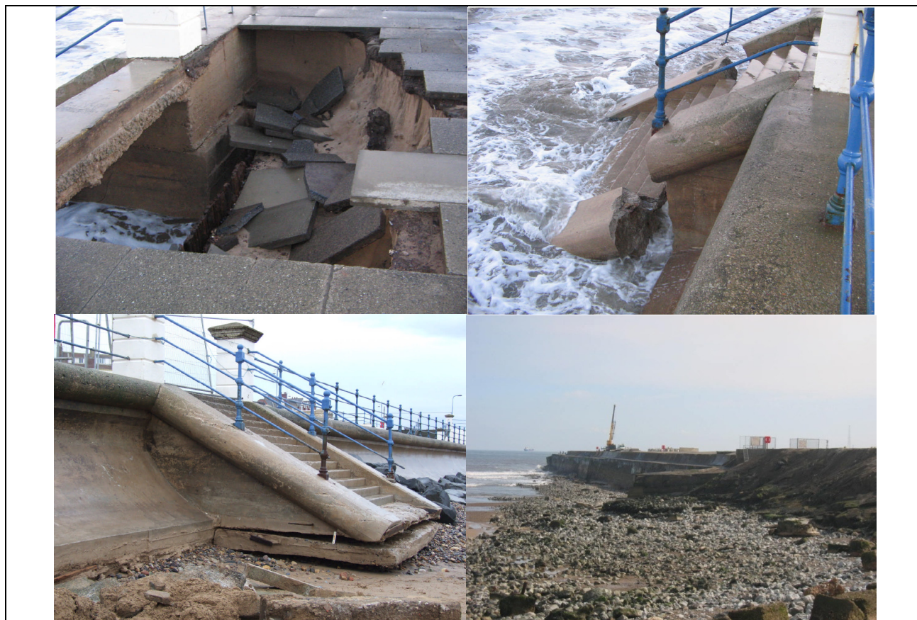
Recent damage sustained by the coastal defences in Seaton Carew and North Gare Breakwater (2003)
