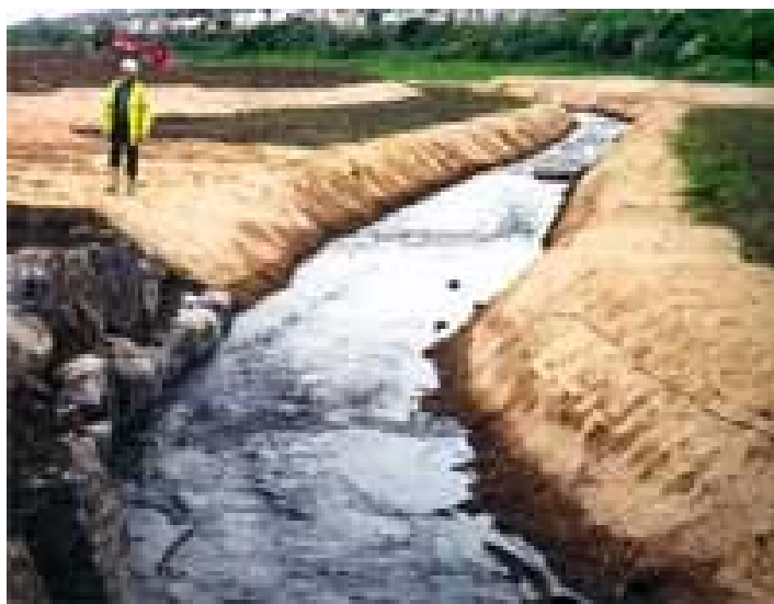
A re-profiling scheme under construction on a small watercourse.
