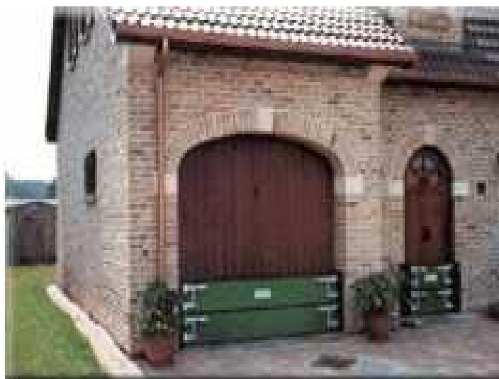
Flood proofing of a residential property.
