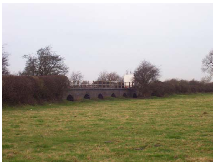
Flood relief culverts under Wellington Causeway allow the passage of water across the floodplain.
