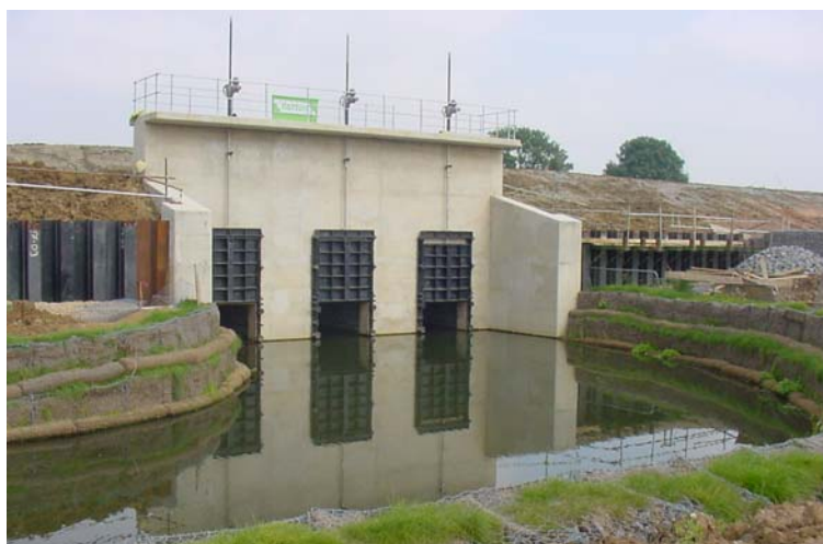
An on-line storage reservoir under construction on a small watercourse; the photograph shows the upstream face of the dam and the control gates, which are used to regulate water flows.
