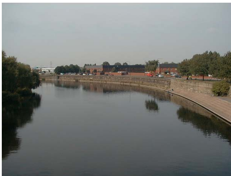
Flood defence walls along the River Trent at Queens Drive, Nottingham.
