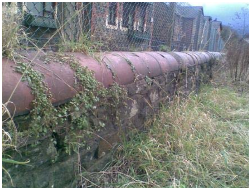
Figure 6 Existing natural stone wall, re-use of the stone will retain the character of the area and save waste.
